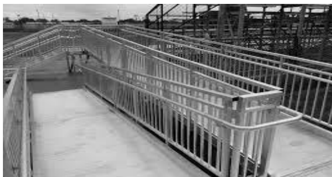
Wheelchair ramp (Image taken from http://stlouis.101mobility.com/wheelchair-ramps-stlouis.php )
